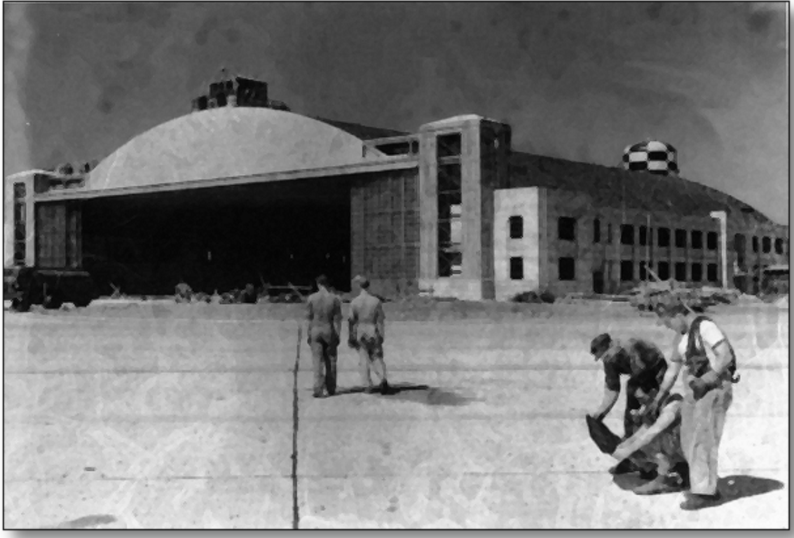
A hangar under construction at MacDill Field in June 1941.
